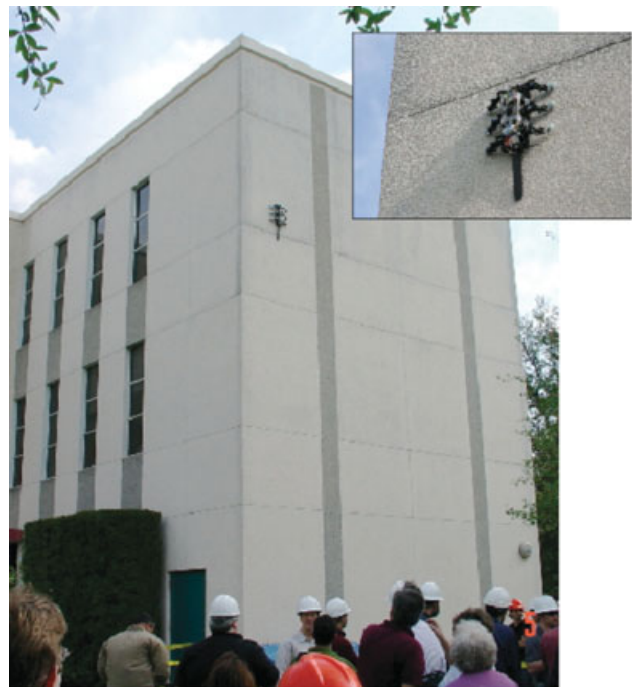
Figure 20. The RiSE robotic platform (view and detail) while completing an untethered climb of a three-story ( \approx 12 m) concrete building, making use of the feedback behaviors described in this paper.
